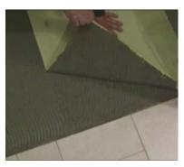
22. Trowel at least 2" wide path of thin-set to prepare for the membrane overlap. Repeat previous process of laying overlapping membrane into thin-set and pressing in with flat end of trowel. Many times throughout the entire kit installation, peel back the membrane to ensure you are achieving 100% thin-set coverage of the membrane. Finalize the overlap installation in this section of the pan floor by pressing and smoothing the overlapping membrane section at the seam.
