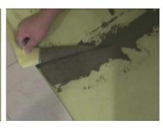
Repeat the installation process on any remaining sections of the pan area until the entire all sections of membrane are completely overlapped at least 2" in every direction and properly seated into the thin-set.
