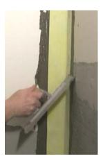
27. With all joints and corners complete, begin to install the wall pieces starting from the bottom up. Ensure at least a 2" overlap on any adjoining sections. Installation continues exactly like it did for floor sections. As always, peel back membrane to ensure 100% coverage and constantly run hands over membrane to feel for any trapped air bubbles.
