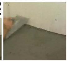
14. For the standard curb form, make your mud mixture a bit wetter and pack the form around the encased and protected 2x4's with this mixture. Then screed the curb smooth. Let the entire mud job dry for 24 to 48 hours.
