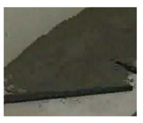
13. Starting at the back furthest from the entrance to the shower, spread and pack the mix fully between and around the sticks with a flat trowel. Using a straight edge, 2x4 or other suitable tool that is large enough to span the
