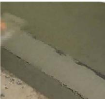
15. For the handicap curb form install, remove the handicap form from its test-fit position and shovel a row of mud along the length of the handicap curb run. Press handicap curb form into mud and into its proper position. Screw down the handicap curb form into position with 1-1/4" screws (Tapcon screws for concrete) subfloors. Fill and pack any remaining voids in the form with additional mud and screed smooth with a trowel.
